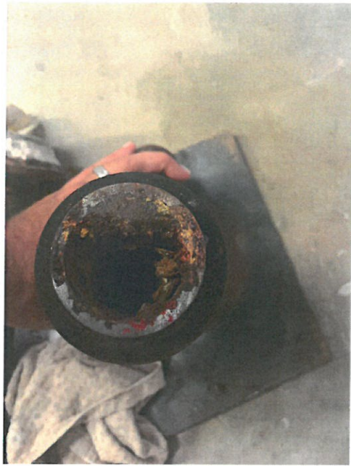
P-Trap Blockage of Unit 4S
