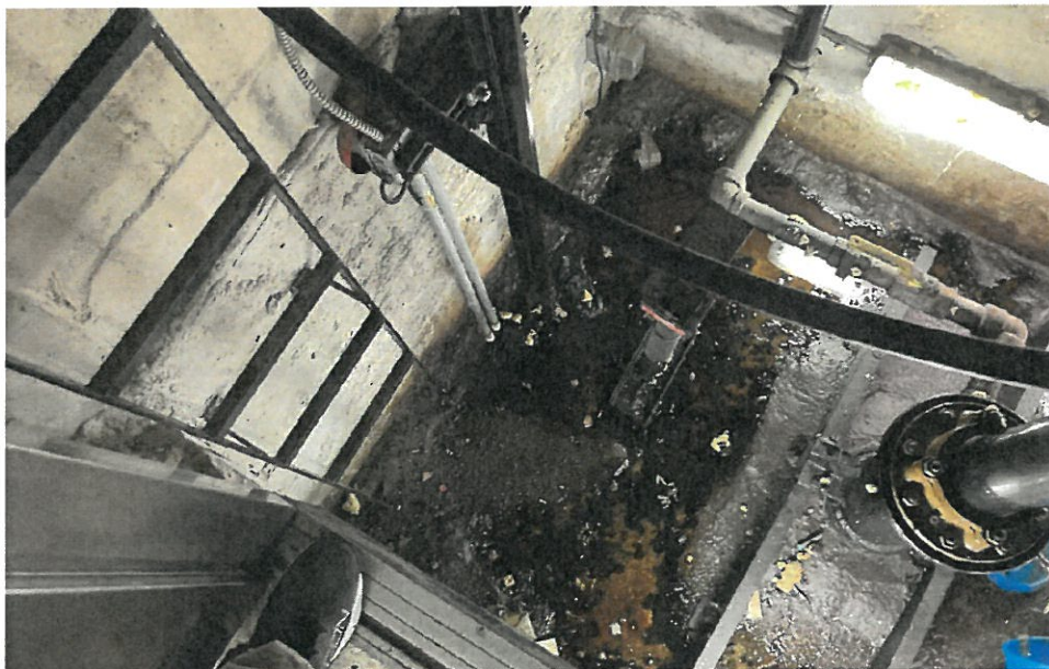
Elevator Pit with Ponding Fluid in Bottom
