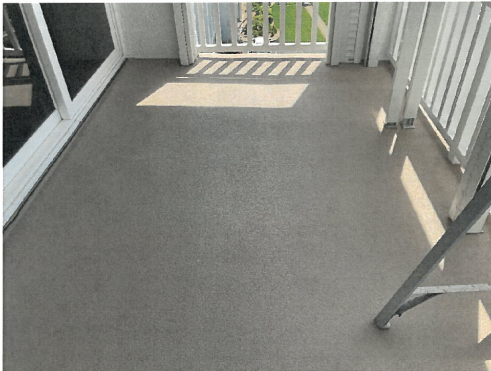
Applied Floor Coating on Balcony
