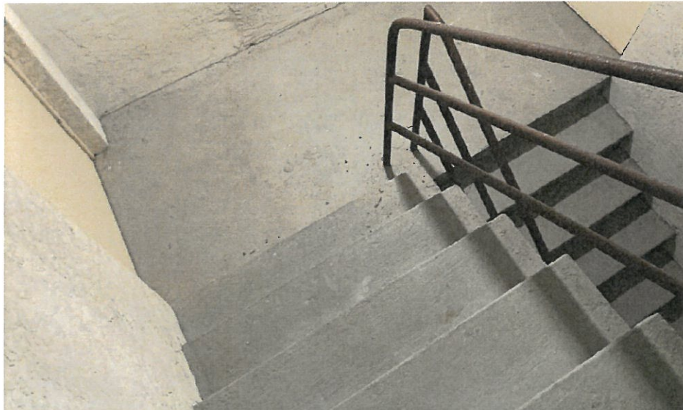
Noncontinuous and Single-side Installation of Railings for Exit Stairwell
