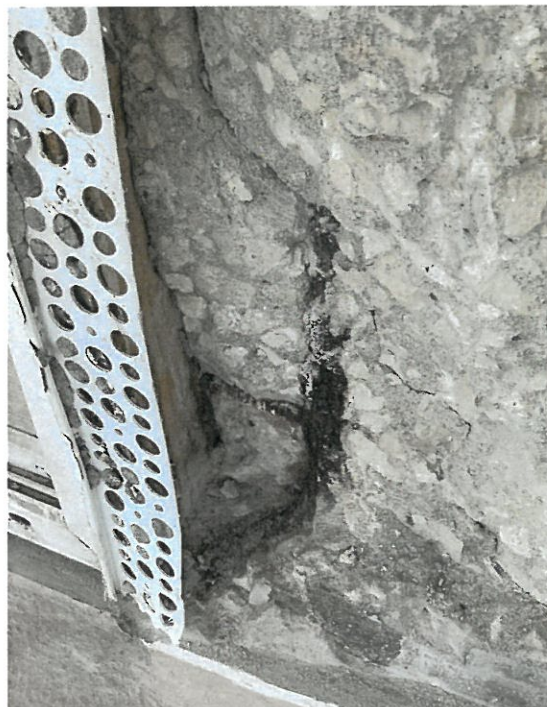
Repair In-Progress of Identified Spall on Unit 4N Column (Taken 2023-02-14, Repair Completed)
