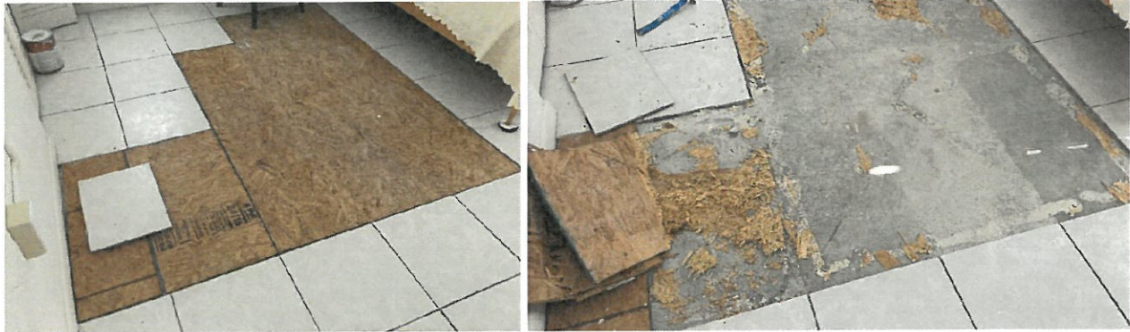
Removed Tile Finishes from Unit Bedroom and Exposed Slab
