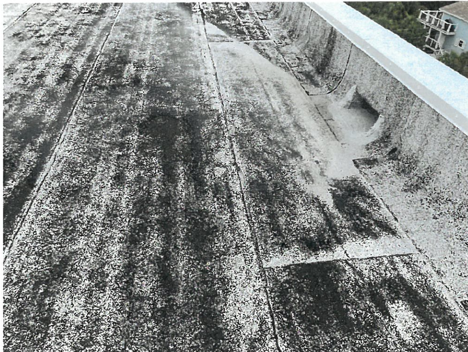
Scupper with Minor Ponding (Scupper Appears to be Above the Sloped Roof)
