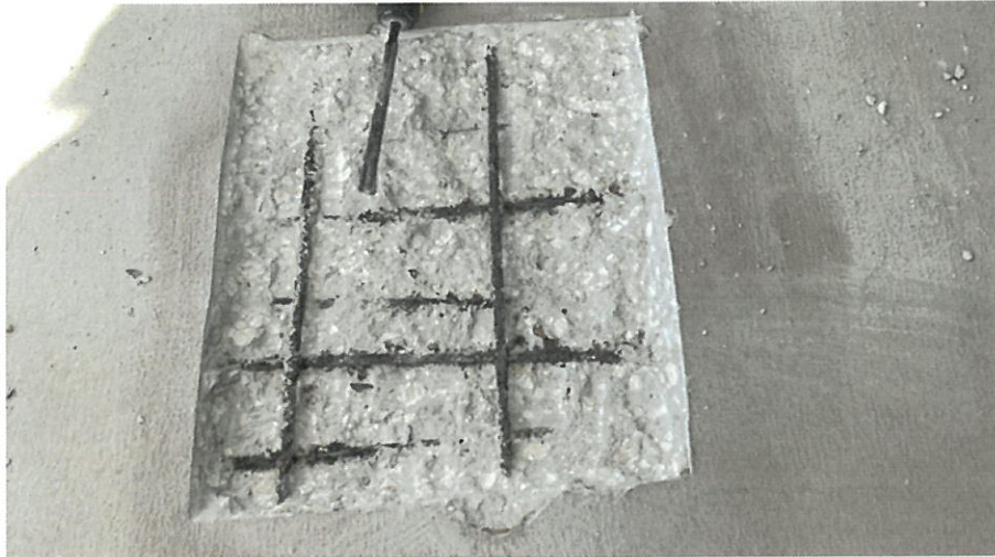
Repair In-Progress of Identified Spall on Unit 2N Balcony (Taken 2023-02-14, Repair Completed)
