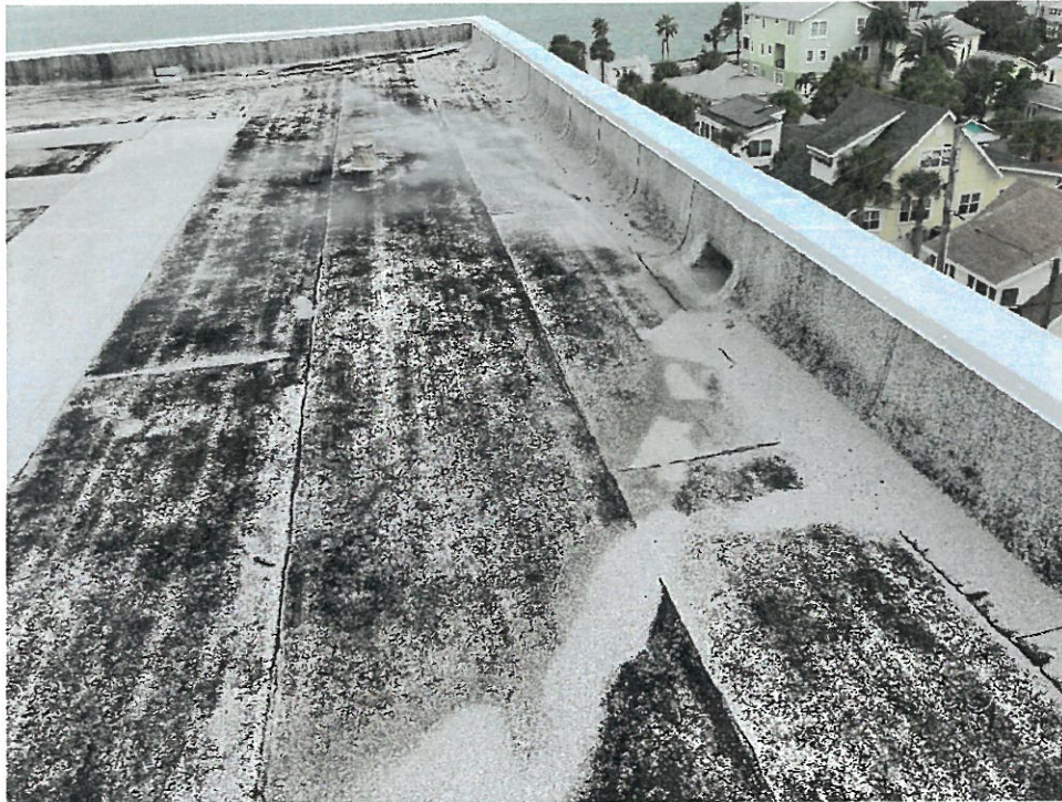
Granule Loss and Ponding on Roof Membrane Surface
