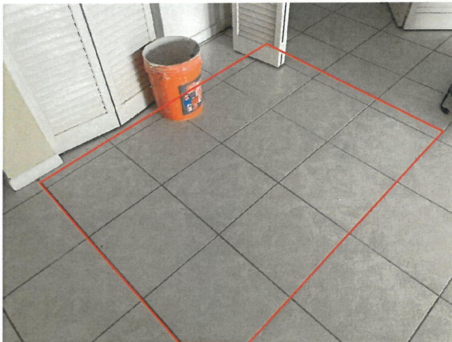
Section of Apparent Debonding Tile Finishes
