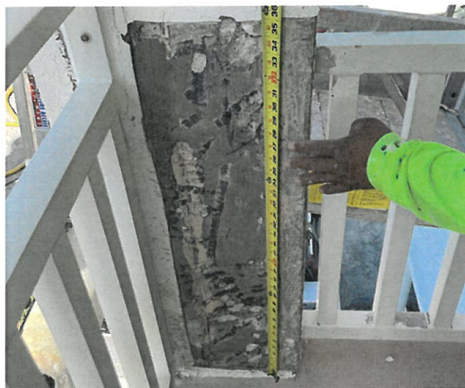
ICCP Protected Column with Repairs Limited to Debonding Stucco Finishes (Taken 2023-02-10, Repair Completed)
