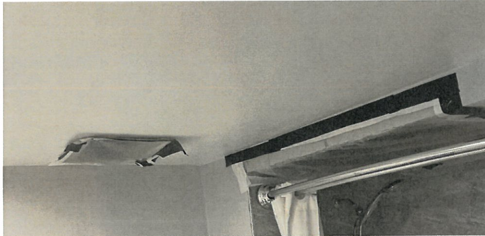
Unit 4S – Bathroom Finishes Damaged due to Leak from Above
