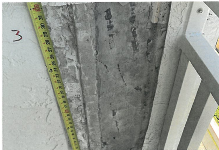
Repair In-Progress of Debonded Stucco (Taken 2023-02-10, Repair Completed)
